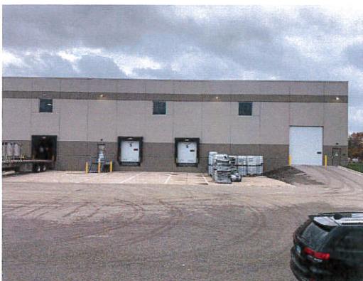
4 A11 EXISTING PHOTO
