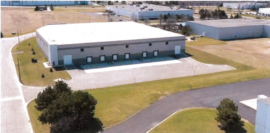
3 A11 EXISTING PHOTO
