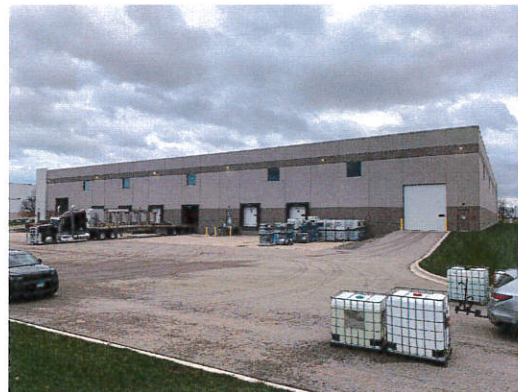
5 A11 EXISTING PHOTO
